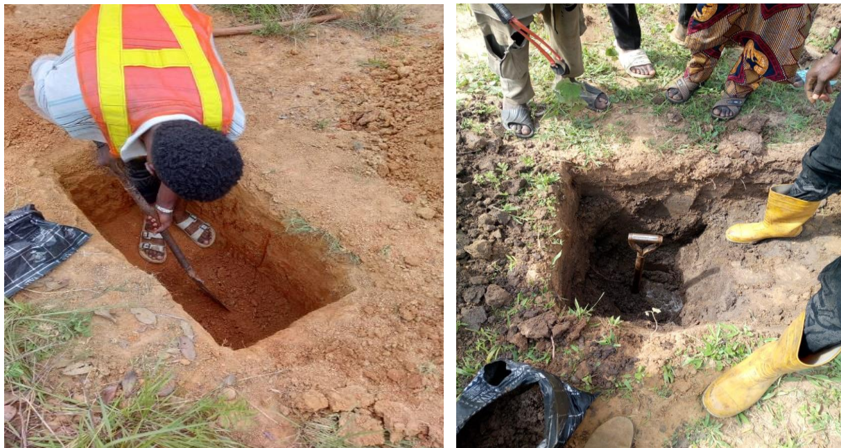
Plate 2: Trial pits for sampling of disturbed and undisturbed samples.
